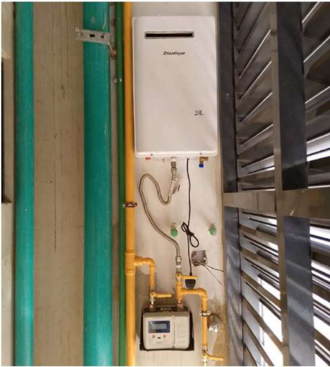
Otentique Gas Water Heater with Gas meters Installed
