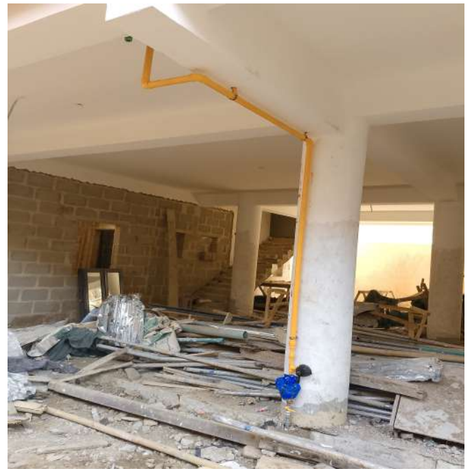
Ongoing Installation at a Hotel in Ohafia, Abia State
