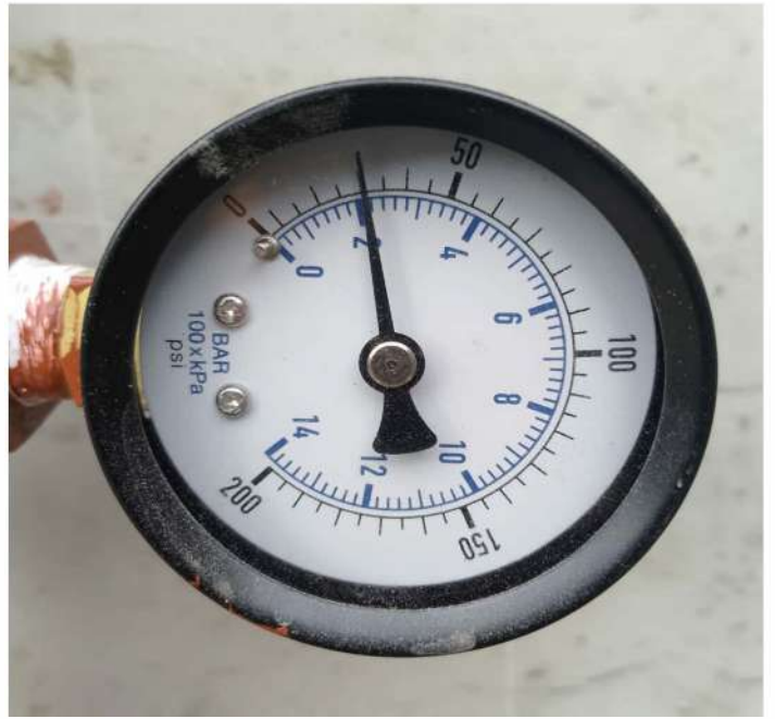
Gas Gauge with gas flowing
