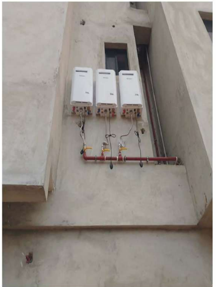
Installed Otentique Gas Water Heaters
