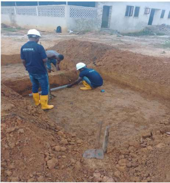
Preparation of Concrete Plinths for Gas Tanks
