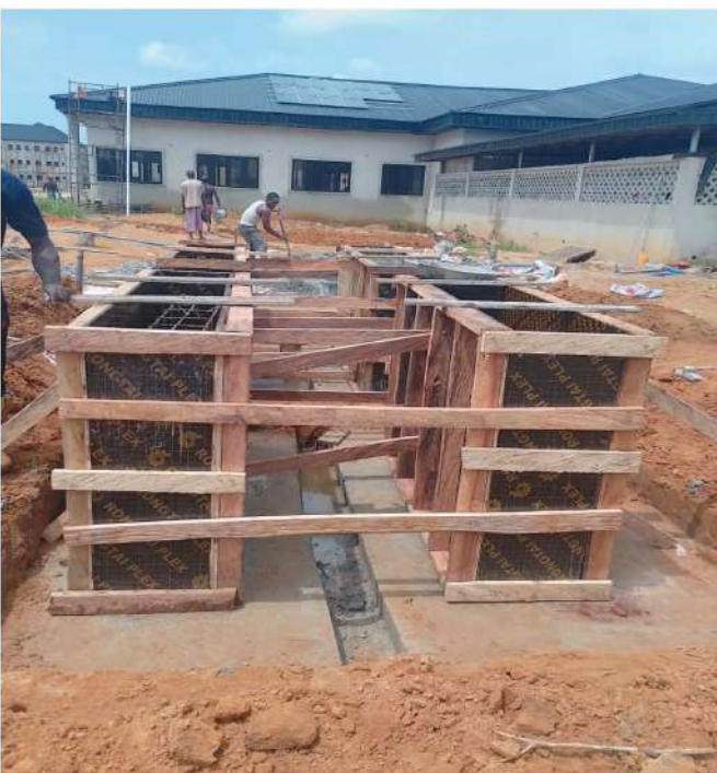
Casting of Concrete Plinths for Gas Tanks
