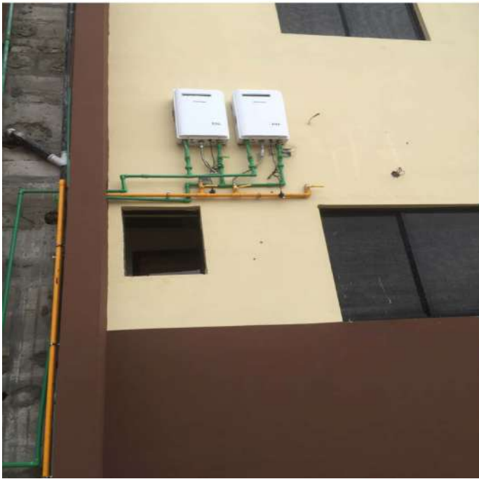
Installed Otentique Gas Water Heaters
