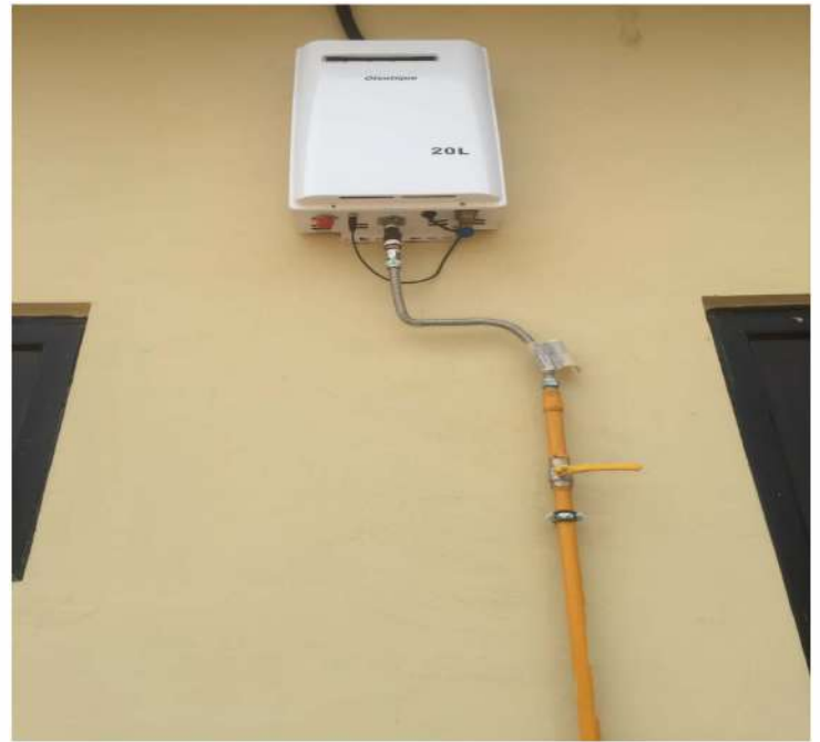
Installed Otentique Gas Water Heaters
