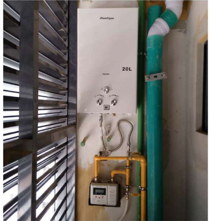
Otentique Gas Water Heater with Gas meters Installed
