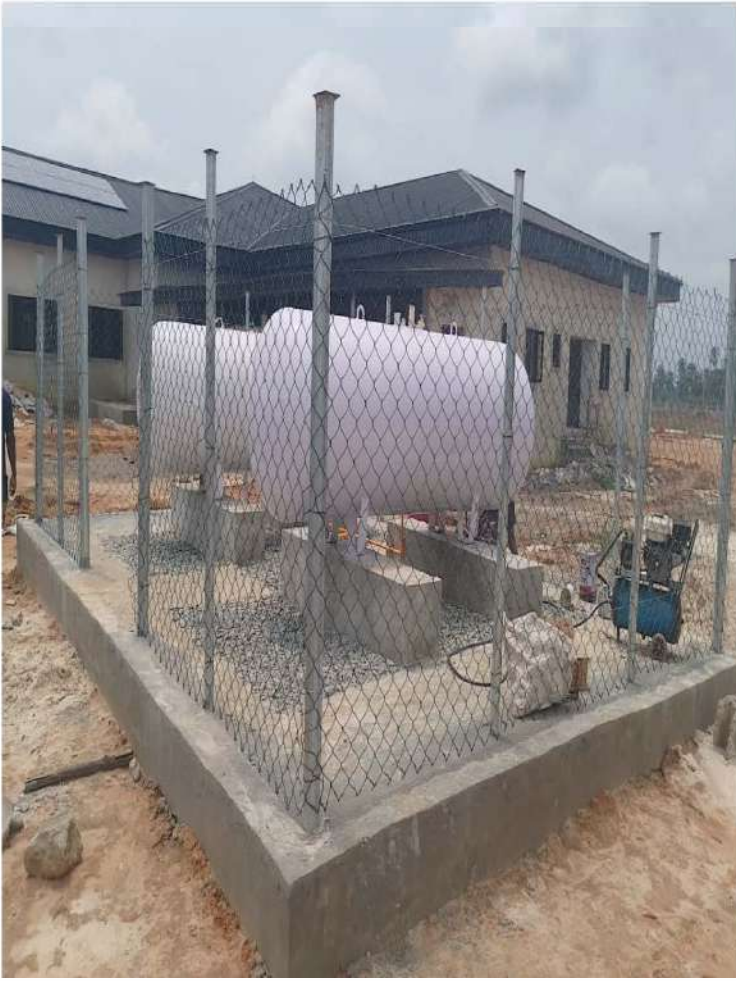
Installation of Gas Tanks
