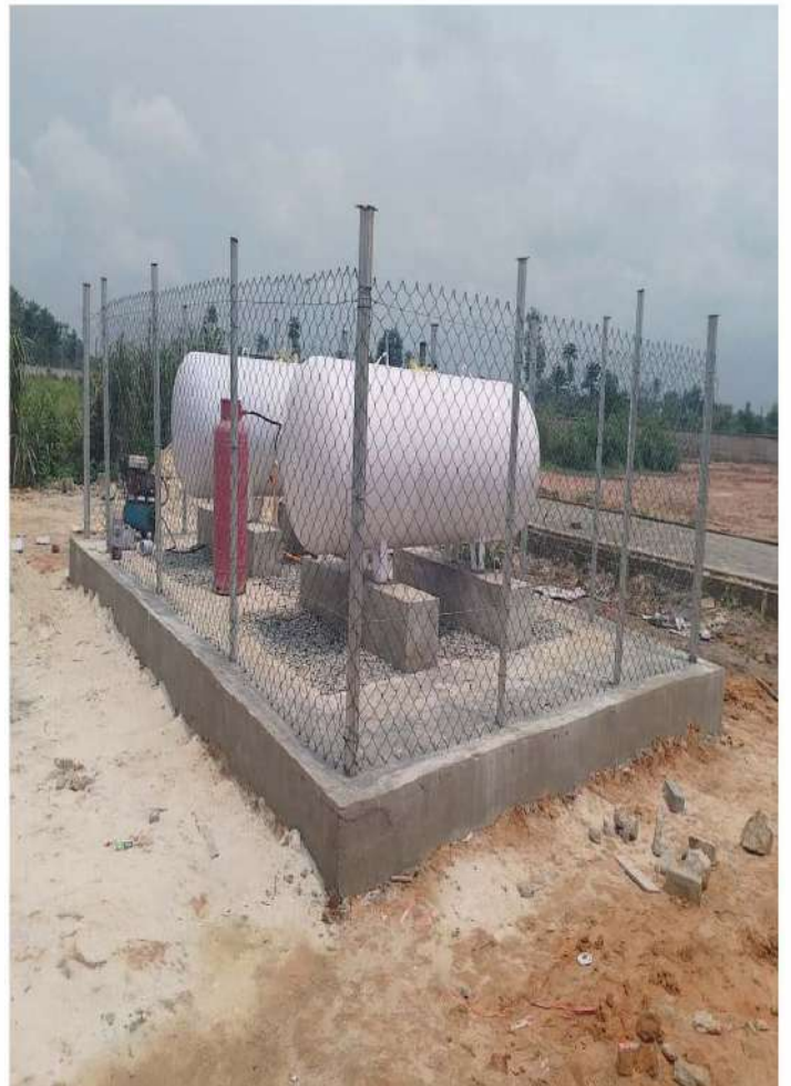
Installation of Gas Tanks
