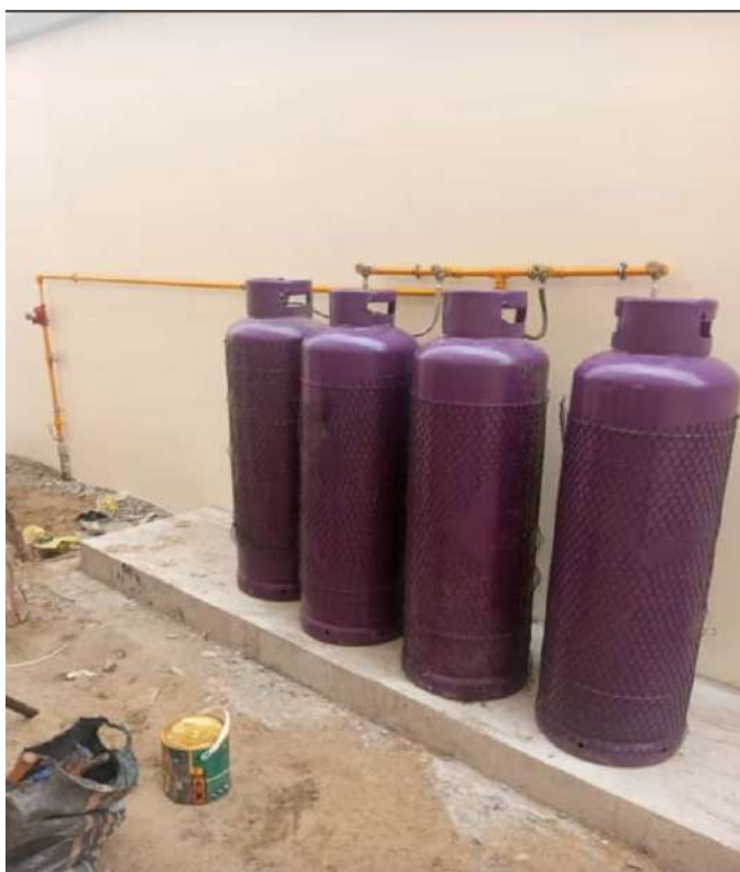
Ongoing Gas Cylinder Manifold Installation
