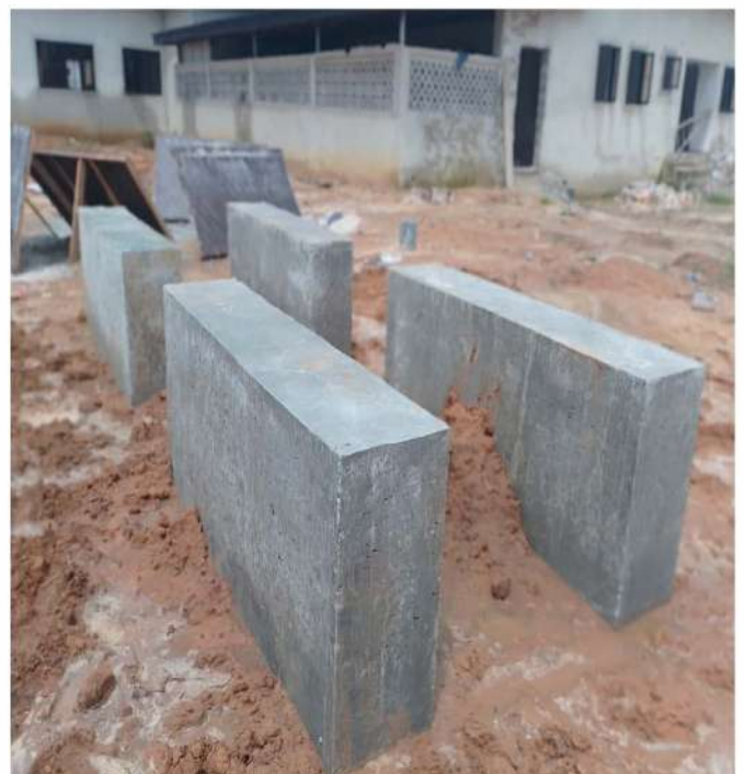
Concrete Plinths for Gas Tanks
