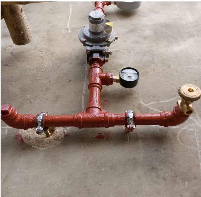
Gas line and Manifold Installation
