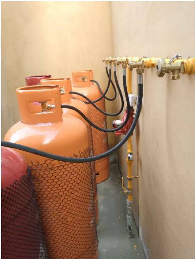
Completed Project with Gas Reticulation and Water Heaters
