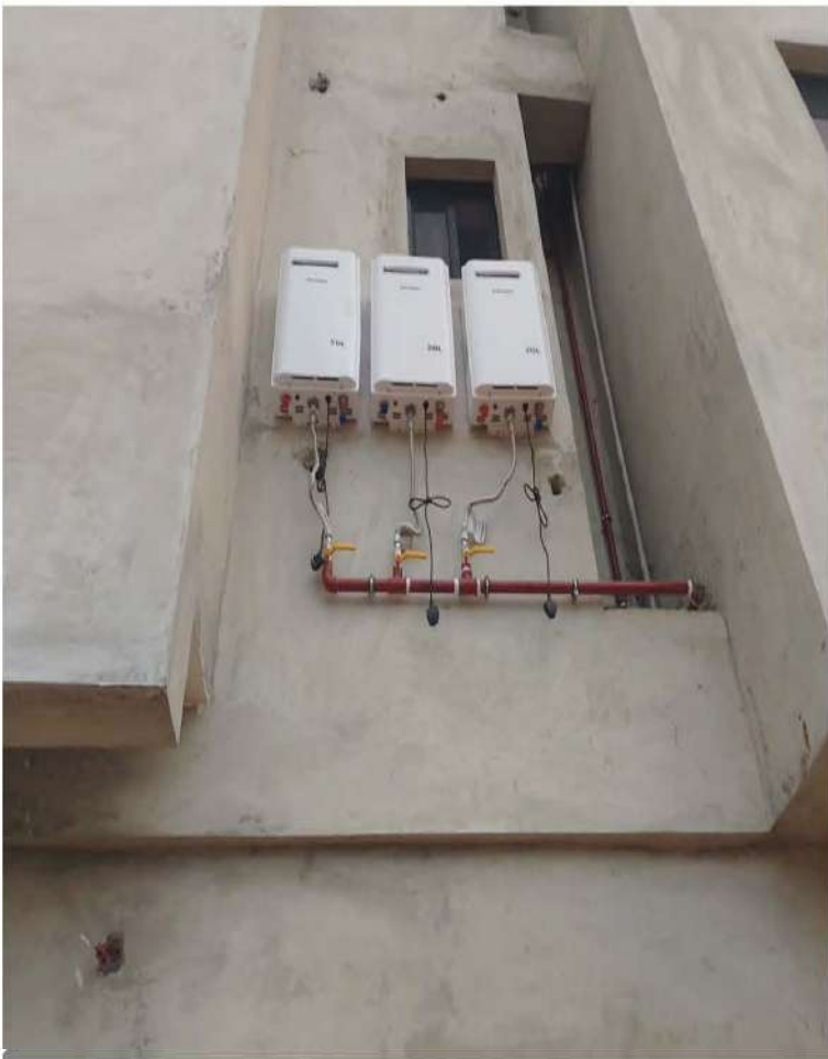
Installed Otentique Gas Water Heaters
