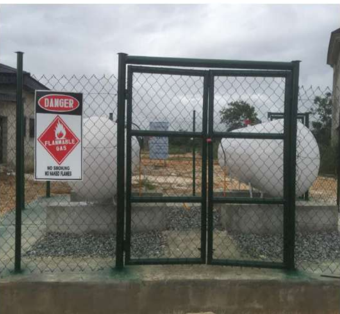
Completed Gas Tank Installation
